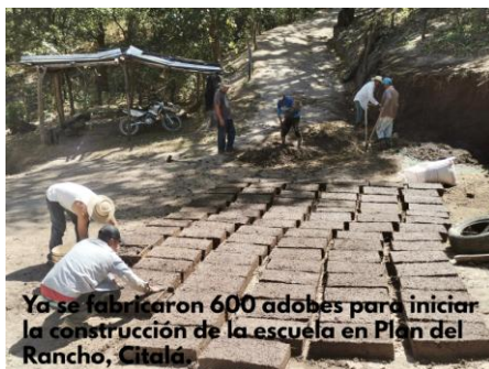
Right: First 600 adobe bricks for school construction
